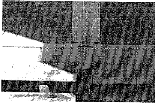
This is a photograph of the exterior deck deflection between units 314 & 316 ?.
