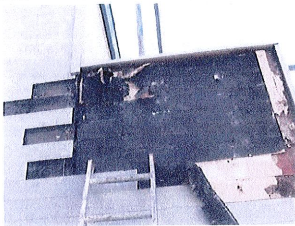
Figure 23: Wing wall built over existing structure
