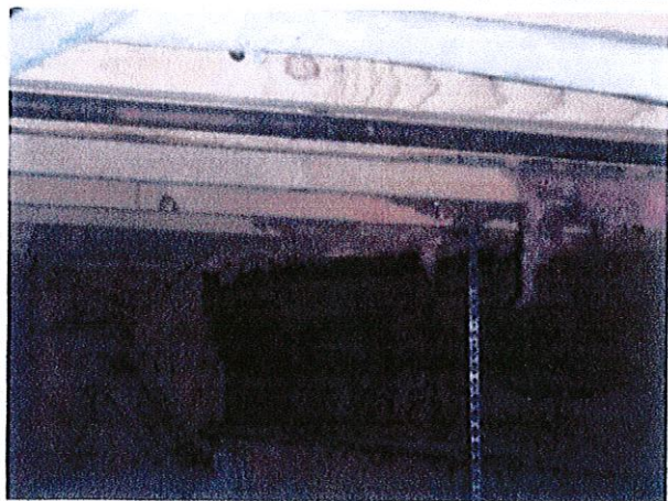
Figure 42: Insulation falling out of floor joists (photo courtesy of REG)
