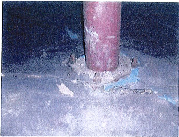
Figure 37: Poly ground cover at lally column
