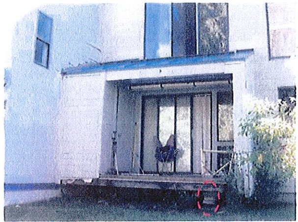
Figure 20: SW porch with added "support"
