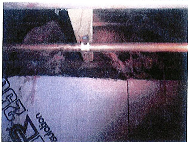
Figure 40: Deteriorating sill plates in 300 building crawl (photo courtesy of REG)
