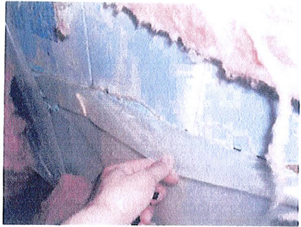
Figure 38: Poly ground cover sealed to wall insulation
