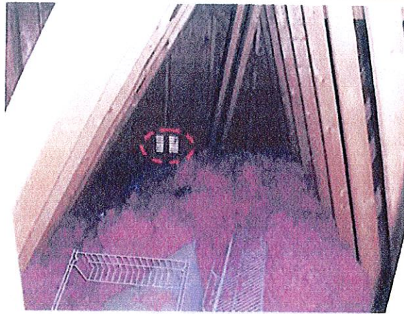
Figure 10: Attic Vent from Interior
