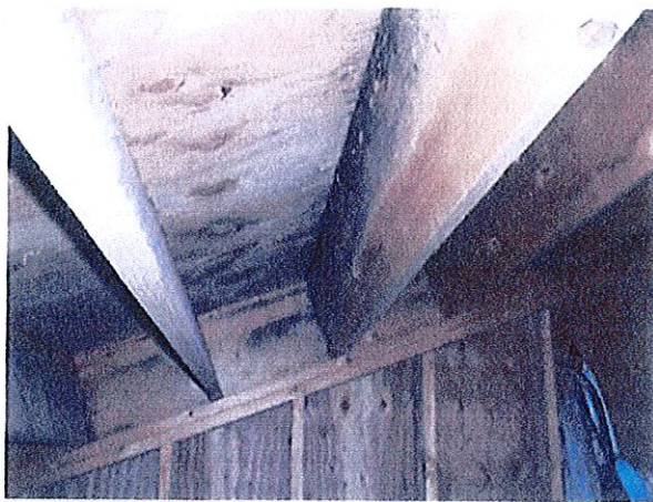
Figure 11: Attic condensation stains
