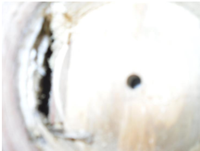
Close up detail of separation of drywall and plywood.
