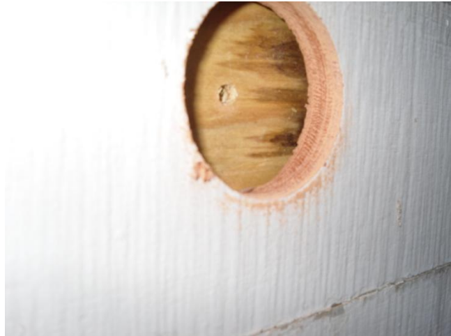
Close up detail of plywood showing signs of moisture.
