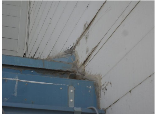
400 South Gutters showing exterior mold.
